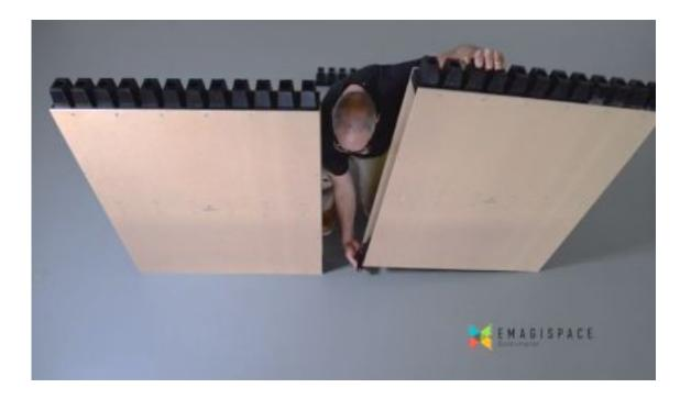
2. Lift the corner of the second Emagiblock® and set it on the second half of the EmagiClip™.
