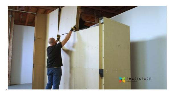
2. Install an EmagiClip™ at the top of the wall to unitize the first and second EmagiBlock<sup>®</sup>s. This EmagiClip™ should be placed over the seam where the two EmagiBlock<sup>®</sup>s meet.
