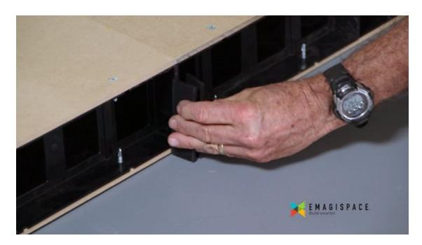
4. Gently tap the EmagiClip™ into place, to secure the blocks to each other.
