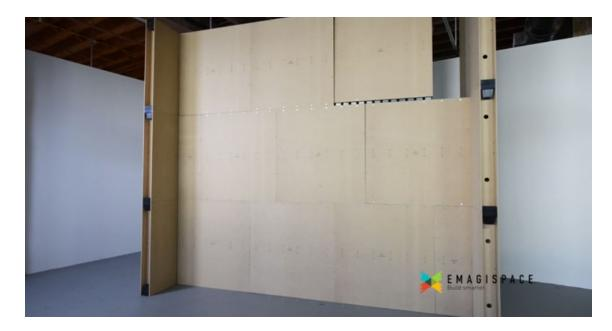
4. Install another EmagiClip™, at the top of the wall, to unitize the second and third EmagiBlock<sup>®</sup>.
