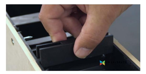
5. Continue placing EmagiBlock<sup>®</sup>s and installing EmagiClip™s on the top course, until the top course of the wall is complete.
