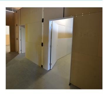
Steel apertures with almost any door mounted inside can be framed or frameless and come in virtually any size. ADA compliant double doors, single hinge doors, Dutch doors... you name it, EmagiBlock®s simply mount around the door.
