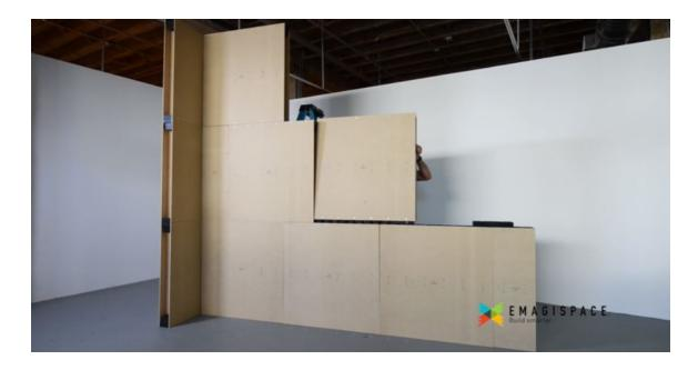
15) Use a Block Connector to temporarily secure this 36" EmagiBlock $^{\circledR}$  to the second course.
