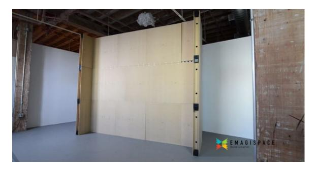
26) Secure the 12" EmagiBlock<sup>®</sup> to the second support wall and ensure that all EmagiBlock<sup>®</sup>s on the third course are secured to each other with connector blocks. Secure the EmagiBlock<sup>®</sup> to the wall by screwing through the two screw holes in the connector block (screw directly into a stud when possible)
