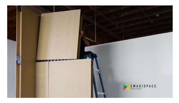
14) Remove the second Block Connector from the top of the first course and place a 36"  $\,$  EmagiBlock  $^{\!(\!R\!)}$  on the second course.
