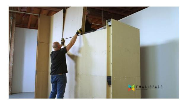
24) Add a third 36" EmagiBlock $^{\circledR}$  to the third course. Place a Connector Block between these EmagiBlock $^{\circledR}$ s to temporarily secure the third course.
