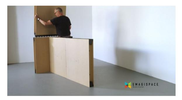
5) Secure the EmagiBlock<sup>®</sup> to the support wall, by screwing through the two screw holes in the connector block (screw directly into a stud when possible. If not possible, use toggle bolts /plate and/or other industry standard methods to insure stability.)
