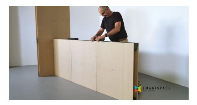
7) Add a 12" EmagiBlock $^{\circledR}$  to the first course and temporarily secure it to the wall with a Block Connector. This is the final piece of the bottom row/course.
