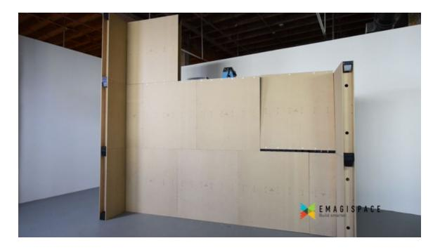
20) Add a third 36" EmagiBlock<sup>®</sup> to the second support wall. Then, secure the 36" EmagiBlock<sup>®</sup> on the second course to the support wall, by screwing through the two screw holes in the connector block (screw directly into a stud when possible. If not possible, use toggle bolts / plate and/or other industry standard methods to insure stability.)
