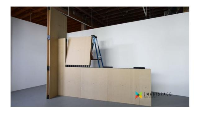
13) Place a 36"  $\rm EmagiBlock^{\it \'R}$  on-top of the second course, flush with the supporting wall.
