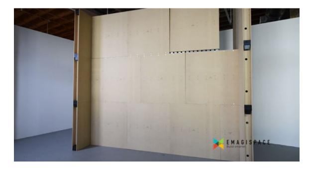
25) Add a 12" EmagiBlock<sup>®</sup> to the third course of the wall. Ensure that the 12" EmagiBlock<sup>®</sup> is flush with the rest of the third course and with the second support wall. Use a connector block to secure the 12" EmagiBlock<sup>®</sup> to the rest of the course.
