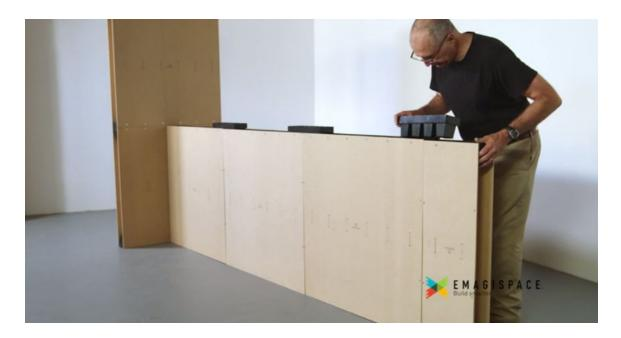
8) Place a 12" EmagiBlock<sup>®</sup> on-top of the first course, and ensure that it is flush with the supporting wall.
