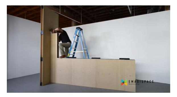
11) Remove the first connector block holding together the first and second 36" EmagiBlock<sup>®</sup>s, on the first course/row.
