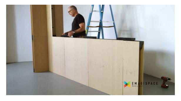
12) Place a 36" EmagiBlock<sup>®</sup> on-top of the first course, flush with the secured 12" EmagiBlock<sup>®</sup>.
