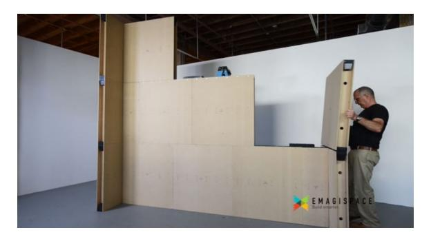
18) Secure the first course of the wall to the support wall, by screwing through the two screw holes in the connector block (screw directly into a stud when possible. If not possible, use toggle bolts / plate and/or other industry standard methods to insure stability.)
