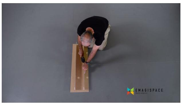
4. Place the second MDF Face Panel on top of the ribs and fully seat the tabs from each rib into the top face panel slots. Make sure the ribs are fully seated in the slots. The blocks should go together fairly easily but sometimes a tab will become misaligned making it hard to seat. In these instances, a slight wiggle will help seat the ribs. Other times, it is possible to use a nail or similar implement to help align the rib tabs with the panel slots.
