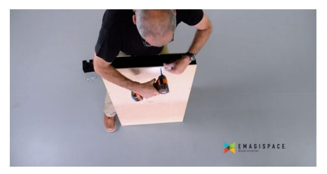
10. Grasp the EmagiBlock<sup>®</sup> on both sides, holding firmly so that the MDF Face Plates stay seated in the Ribs, and carefully flip the EmagiBlock<sup>®</sup> 180° (*Set the EmagiBlock<sup>®</sup>* on the end with the installed BLOCK CONNECTORS, and pay careful attention to keep all the Ribs seated throughout this process.)
