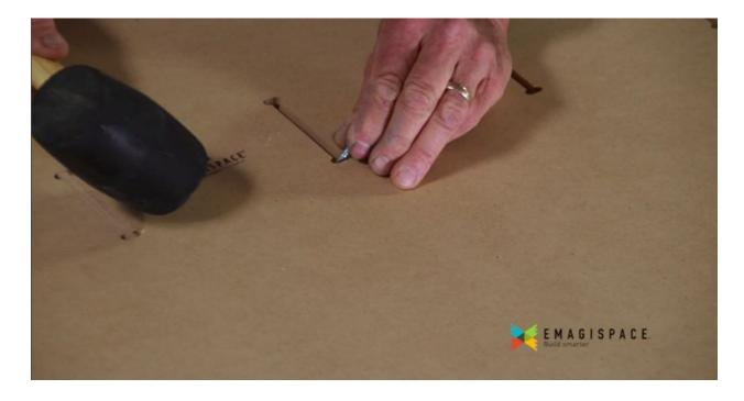
Note: It is always best to work from one side to the other, partially seating the tabs until all are seated. Once all the tabs are seated in the face panel slots, gently tap with your hand or use a rubber mallet to fully seat the tabs in the face panel.
