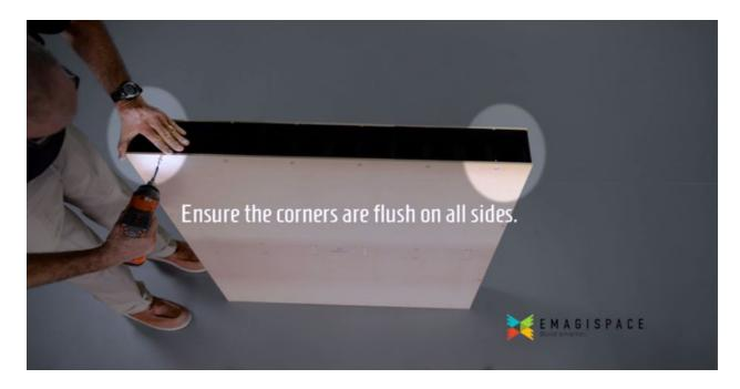
9. Work clockwise from right to left securing all the remaining screws and making sure the BLOCK CONNECTORS remain flush with the corners and edges.
