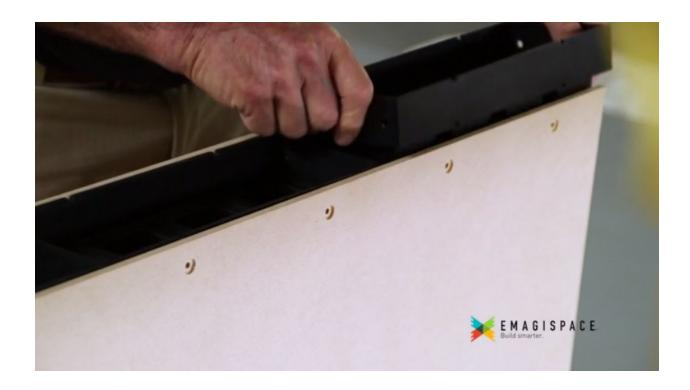
VERY IMPORTANT: BE SURE THE FACE PANELS AND CONNECTOR BLOCKS ARE FLUSH AT THE CORNERS AND EDGES. ALSO, MAKE SURE THE CHANNEL CUTOUTS ARE FLUSH WITH THE RIBS. This seats the Face Panel and prevents the BLOCK CONNECTOR corners from slipping out of square.
